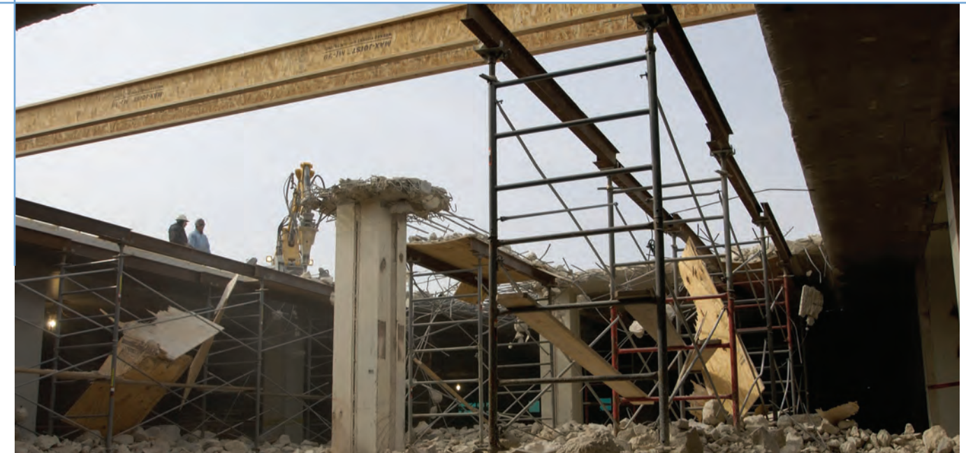
Deconstruction commenced on Technology Business Center 1 this winter.
